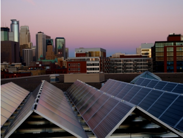
Fig. 4. Non-tracking LCPV design with 3M Cool Mirror (photo courtesy of Ray Colby with Sundial Solar).
